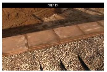
$\label{prop:continuous} {\sf Run\ a\ string\ line\ for\ accurate\ wall\ alignment\ when\ setting\ the\ caps.}$
