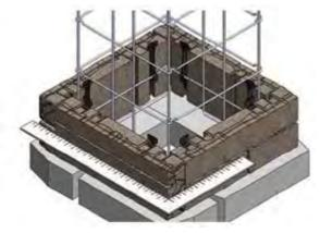
Once you have completed the first two rows, use a square to make sure the column is square and then fill the space with 3/4 " clear aggregate. Fill the empty space with agregates at every row.
