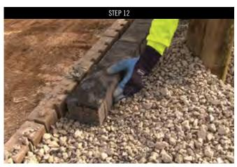
Place a concrete paver directly behind the wall panel and level from front to back. Then take the construction adhesive and place the glue on the paver and top of wall panel. Then secure the cap units to create the bond.
