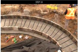
Laying out the radi. Insert plastic connecting members into the veneer dovetails to keep the connectors as straight as possible. Make sure that each veneer has at least two connecting members for proper panel support.
