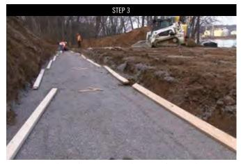
Forming up to pour a 2" unreinforced concrete overlay for setting the first course of Mega-Tandem<sup>TM</sup> Pouring the leveling pad with a low psi concrete. (MSRW). A 6" crushed stone leveling pad is an option as well.
