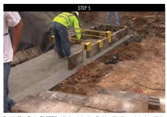
Start the Mega-Tandem<sup>TM</sup> (MSRW) at the lowest elevation. Start by setting the panels in place with the use of the wall jigs to help support the panels during the wall installation.
