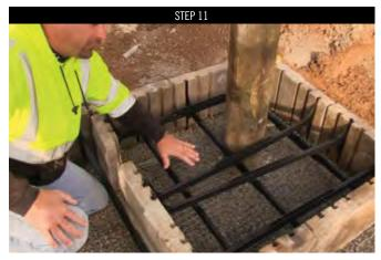
Start the corner with the side textured fitting up against a MT wall (MSRW) panel facing the outer side of the wall. Then place additional panels to create a corner column. Insert the first two connectors upside down for the panel supports (break off the setback tab for this step). Then place two connectors in the opposite direction right side up to support the additional panels. Mega-Tandem Wall<sup>TM</sup> requires four connecting members per course.
