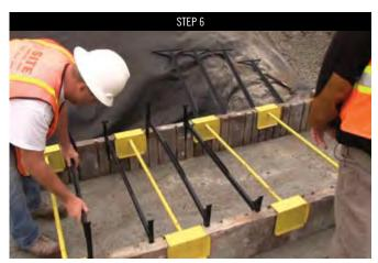
Insert the Mega-Tandem  $^{\text{TM}}$  (MSRW) connecting members into the center dovetails to provide the structural support in the wall system.
