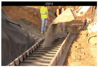
Place the #57 stone inside the Mega-Tandem<sup>TM</sup> (MSRW) panels to provide the internal gravel interlock. This will also provide for internal drainage to relieve hydrostatic pressure in the wall.
