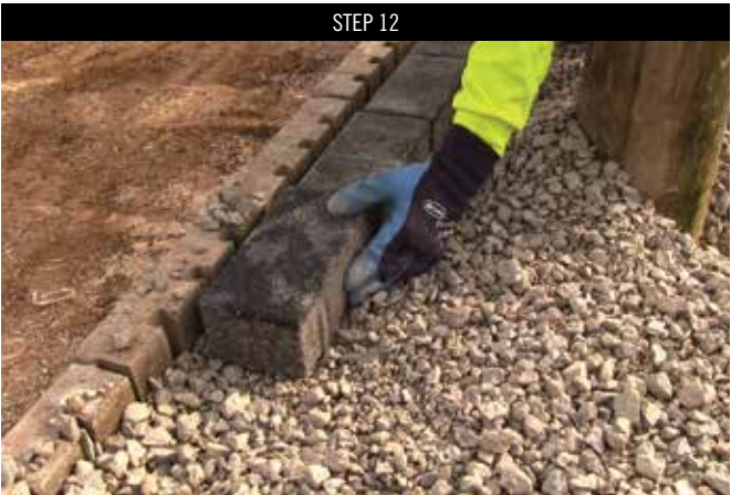
Place a concrete paver directly behind the wall panel and level from front to back. Then take the construction adhesive and place the glue on the paver and top of wall panel. Then secure the cap units to create the bond.
