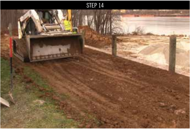
Place a low permeable soil for fill placement for the top of wall.
