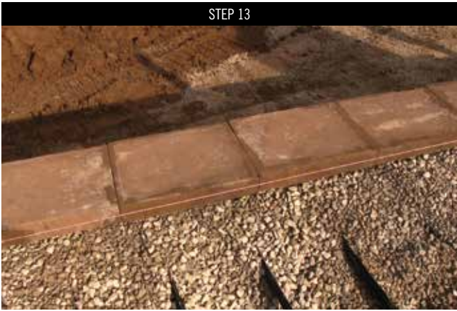
Run a string line for accurate wall alignment when setting the caps.
