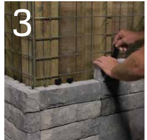
3 Attach Tandem Veneer with Connector
