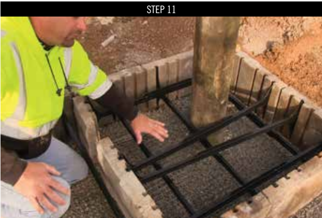
Start the corner with the side textured fitting up against a MT wall (MSRW) panel facing the outer side of the wall. Then place additional panels to create a corner column. Insert the first two connectors upside down for the panel supports (break off the setback tab for this step). Then place two connectors in the opposite direction right side up to support the additional panels. Mega-Tandem Wall™ requires four connecting members per course.
