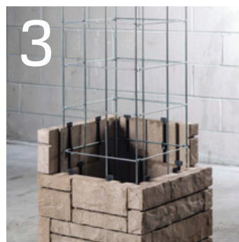
3 Repeat step 2 and fill with 3/4" crushed rock until column is complete
