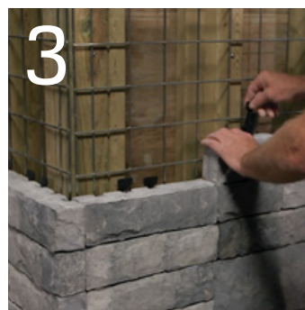
3 Attach Tandem Veneer with Connector
